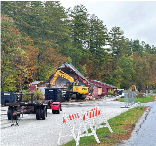
LUDLOW, Vt. – Sam's Steakhouse, in Ludlow, was demolished on Sept. 28. The building was bought out by FEMA after extensive flood damage. Further work continues as
