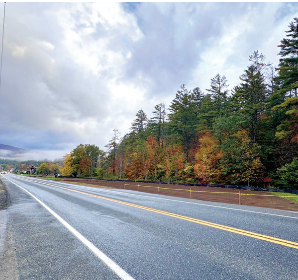
crews cleared the debris and leveled the lot, which will be maintained as a flood plain area. PHOTOS BY SHAWN TAE WEBB
