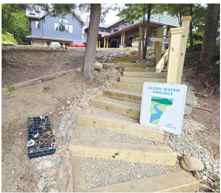
New infiltration steps installed. PHOTO PROVIDED
