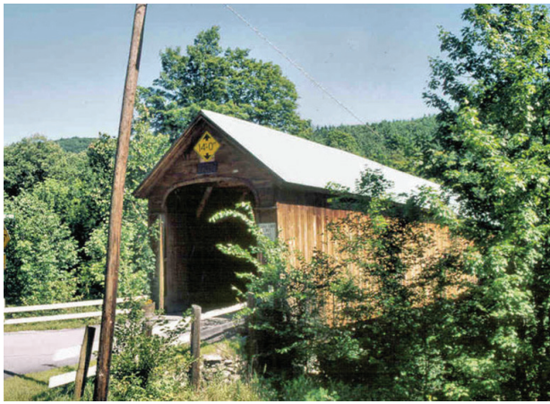
The Hall Covered Bridge, situated on the Saxtons River.
