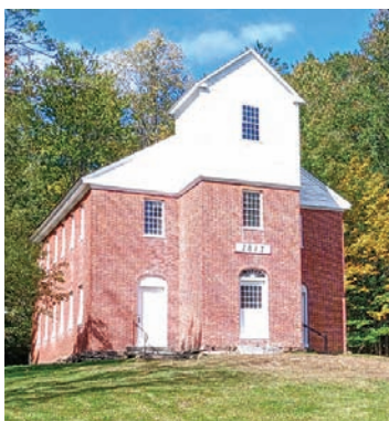
The Athens Brick Meetinghouse. PHOTO PROVIDED
