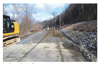
Workers with Casella Construction continue repairs on Route 12 south of Charlestown after having removed the asphalt and concrete base in the damaged section of the road. PHOTO BY CHRISTOPHER SHABAN, EAGLE TIMES STAFF
