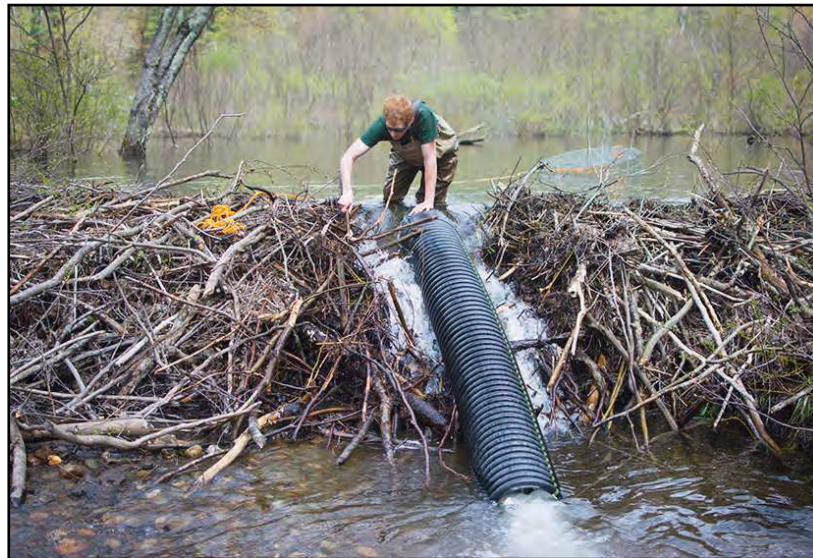
Technician Tyler Brown installs a beaver baffle on a beaver dam in Bolton. The baffle controls water levels to eliminate damage to a nearby road while maintaining the wetlands.
