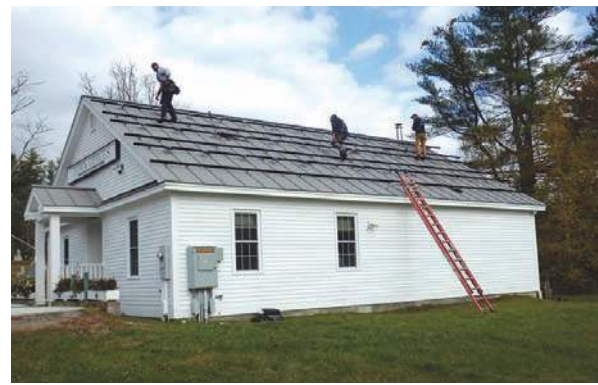
Solar array installation on top of Windham town offices. PHOTO PROVIDED
