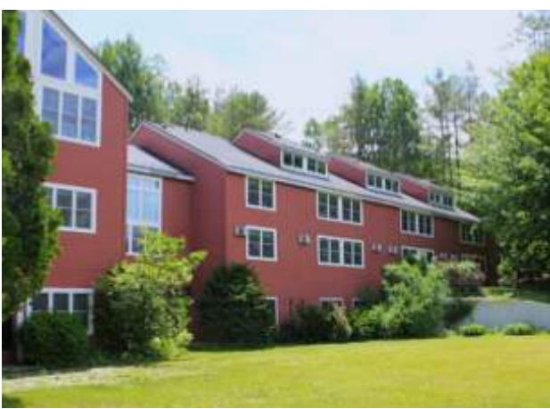
Divided Sky facility.
