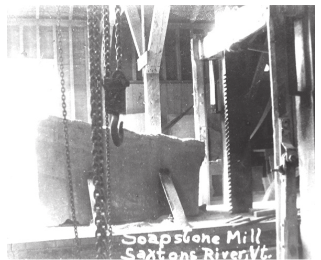
Soapstone Mill in Saxtons River. Notice saw at right. PHOTO PROVIDED BY RON PATCH
