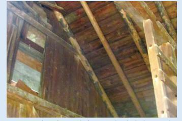
Spruce trees for rafters. Right foreground is the built-in wooden ladder. Notice round rungs replaced with boards.
