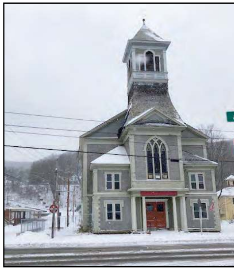
Temporary fencing surrounding the side of 66 Atkinson St.
