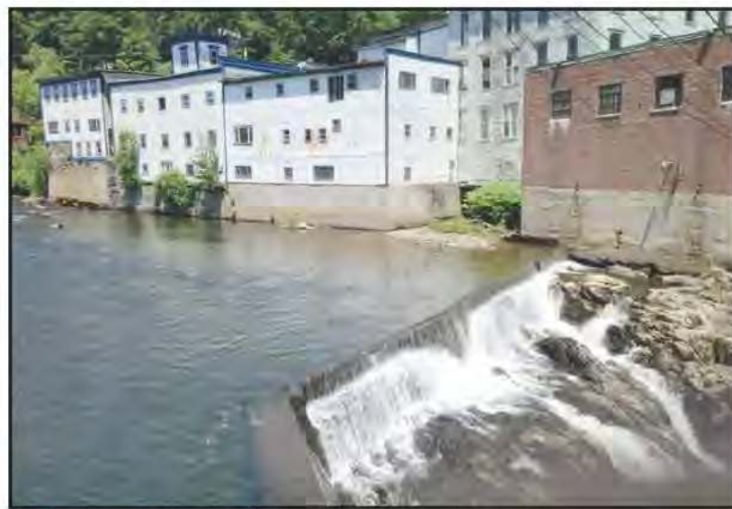
VNA building as seen from Park Street bridge, where the River Walk will be. PHOTO BY KAREN ENGDAHL
