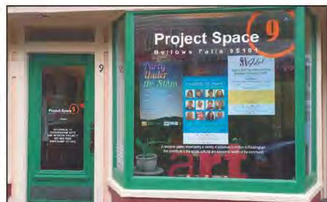
Project Space 9 in the Exner Block.
