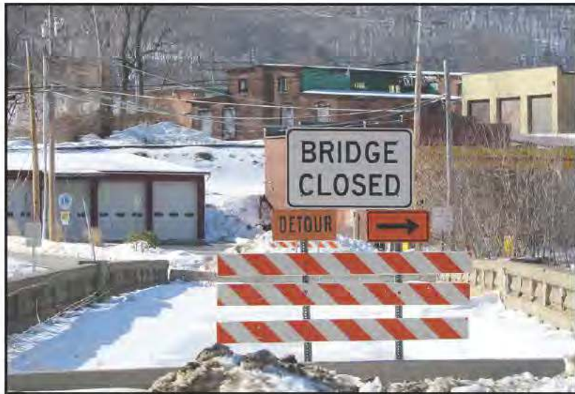
Vilas Bridge entrance.
