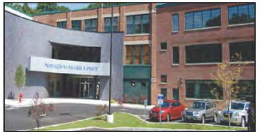
Springfield Medical Care Systems (SMCS) has installed a solar hot water system at its Springfield Health Center location. PHOTO PROVIDED
