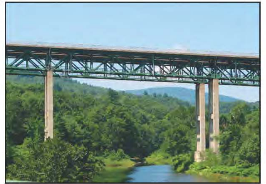
I-91 bridge over the Williams River near Rockingham.
