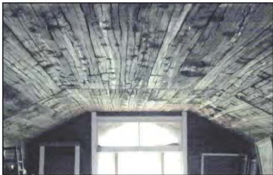
Attic showing lath boards on the ceiling.
